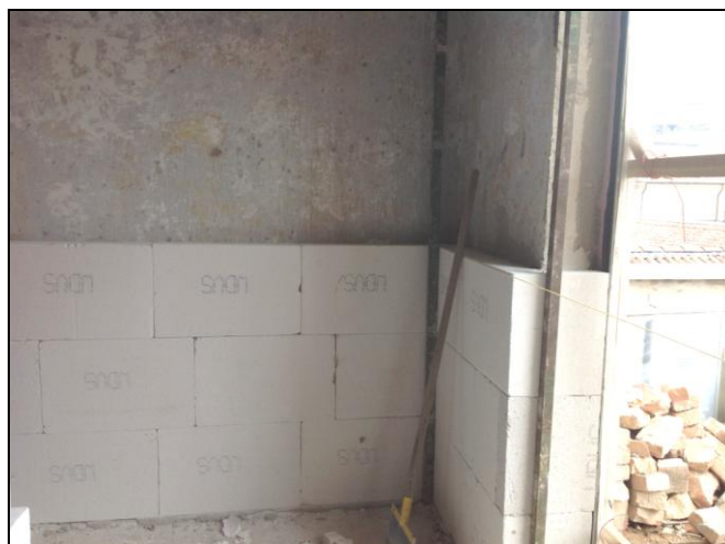
Posa in opera.
